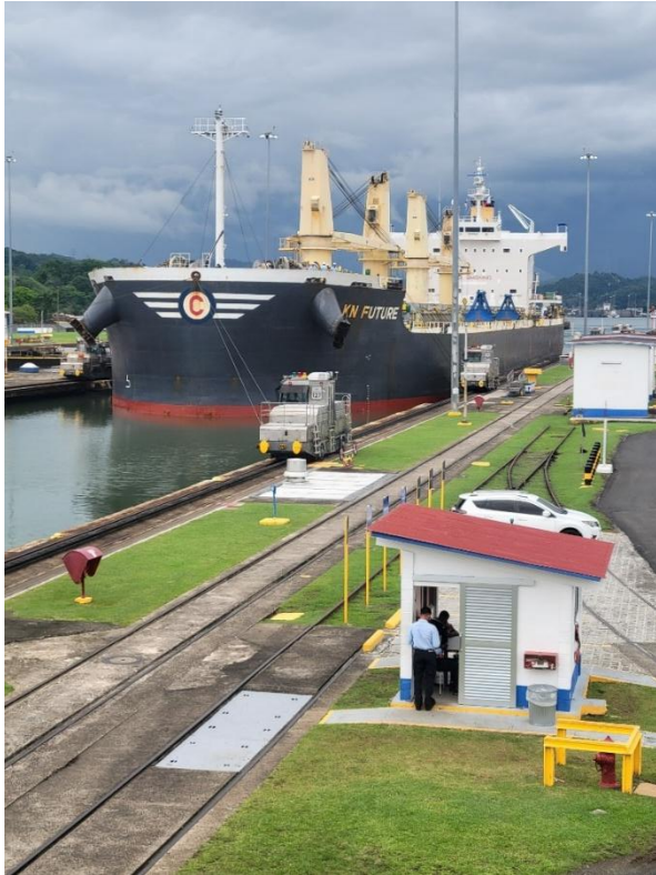
The large ship is moving into position so the back locks can be closed. The ship has stopped and the lock gates behind it are closing.
